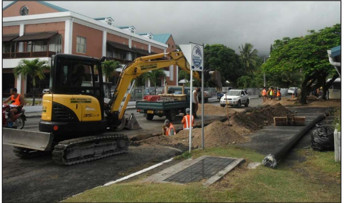
Project City - Mechanically screened removed soil before covering the pipes
